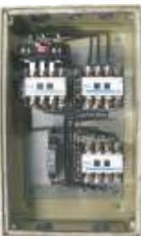
Interior View of MU FASD
