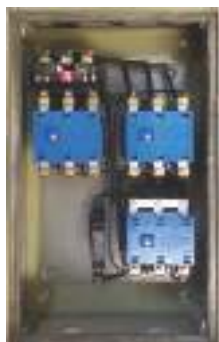
Interior View of ML FASD
